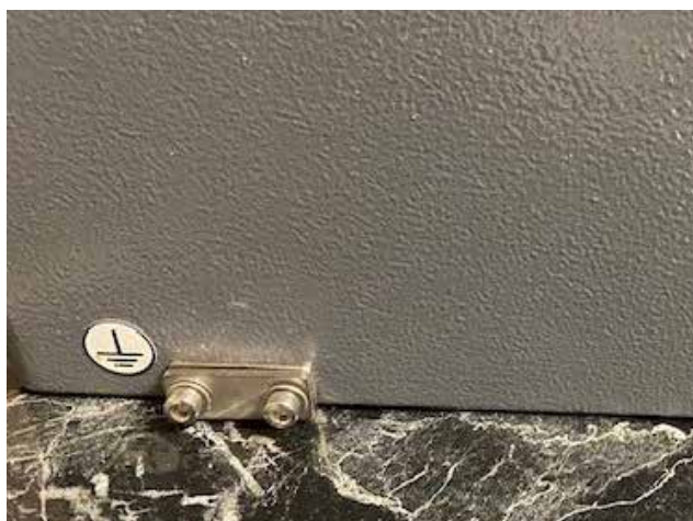
External Grounding Connection Point
